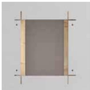
Cut a 225 x 192 x 65 mm rectangular hole in the wall and install 2 wooden planks
